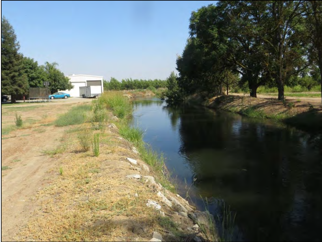
Figure 5. Canal, downstream of the bridge, facing south
