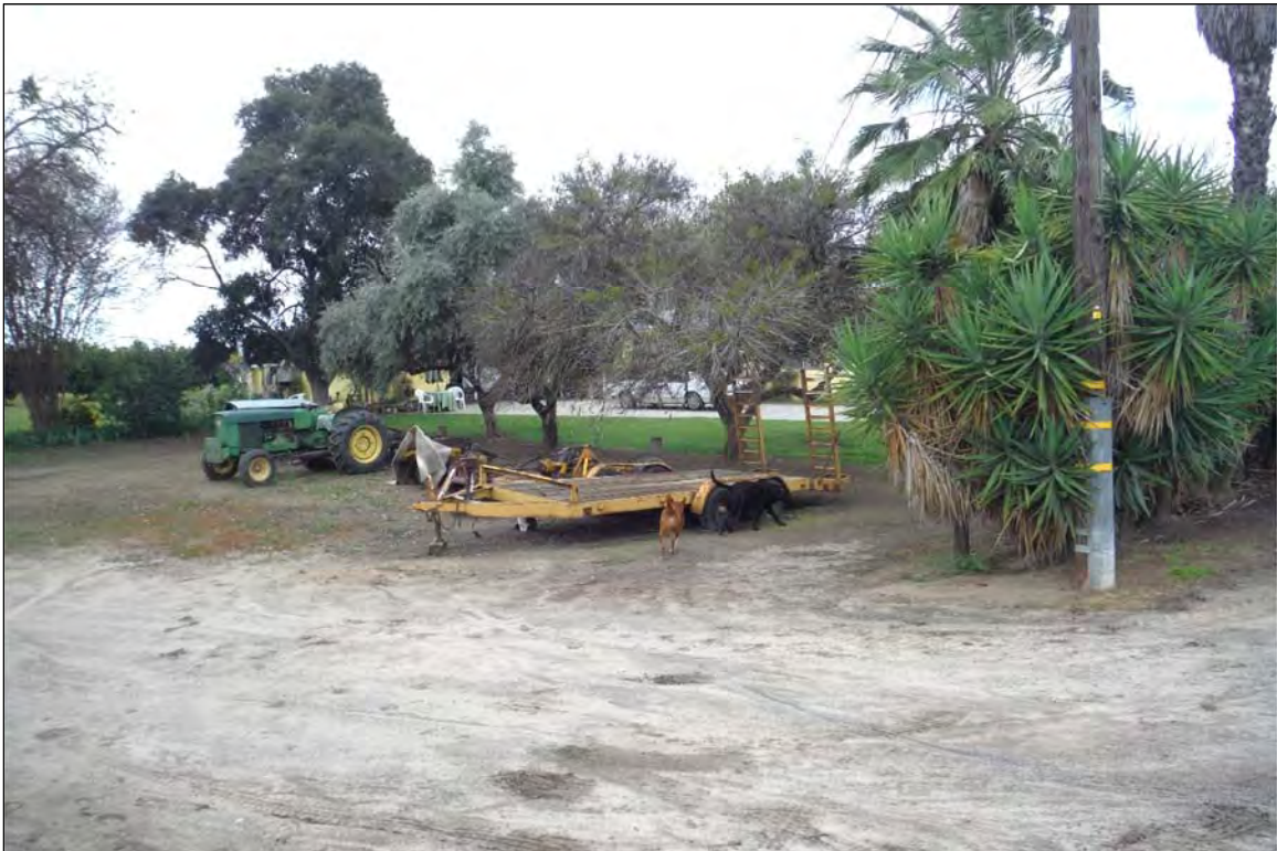
Figure 7 Survey conditions along the southwestern quadrant of the APE; view of the temporary construction easement facing southwest.
