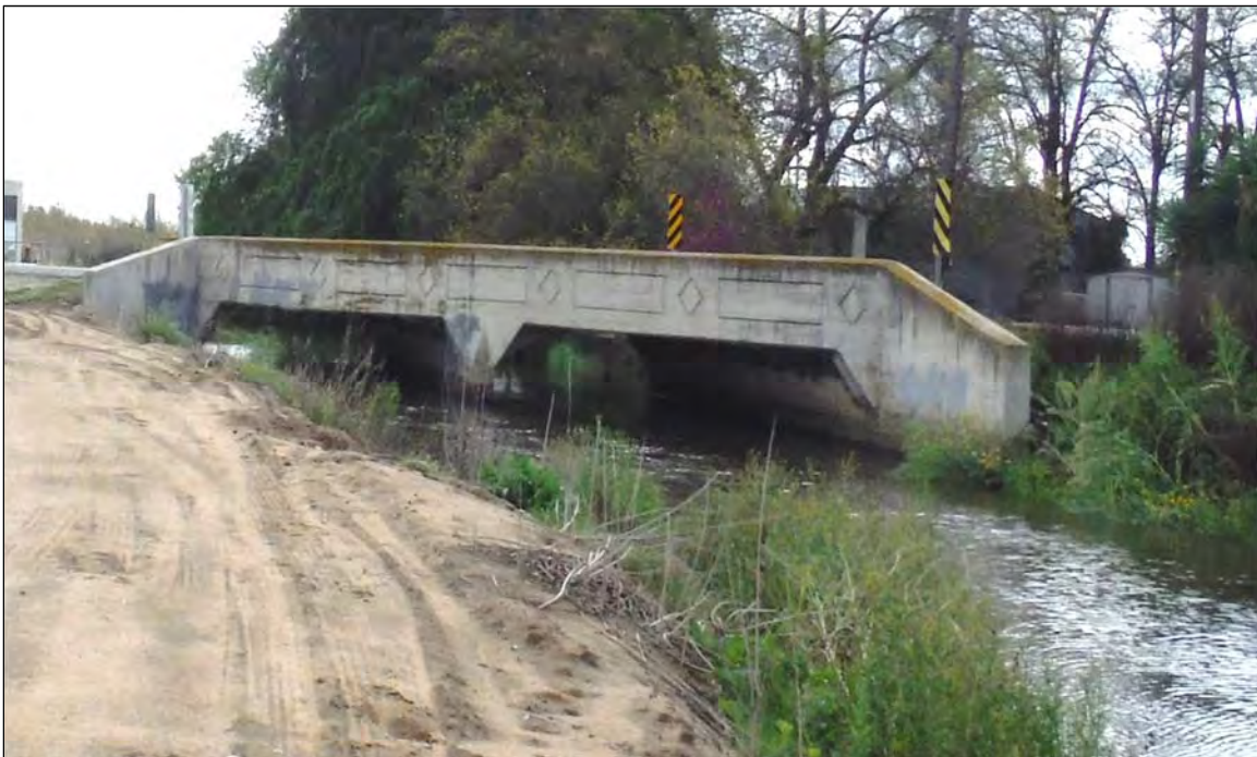
Figure 8 Overview of Bridge 46C0219 from the north, facing south-southeast.
