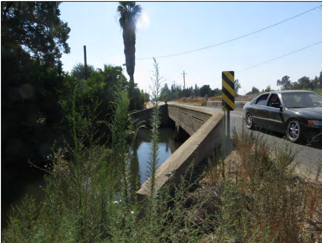
Figure 6. Bridge, downstream, facing west
