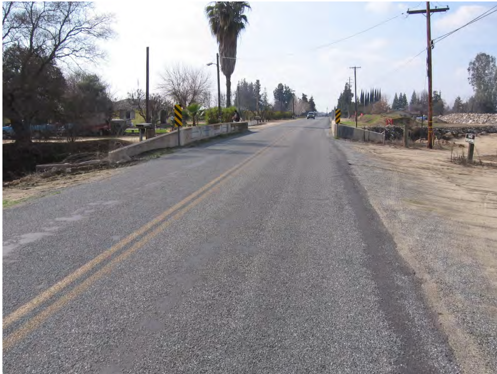
Photo 2. Avenue 424 Roadway Approaches, Looking West
