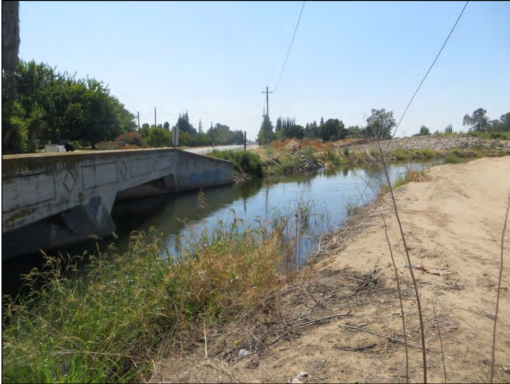
Figure 1. Bridge and Canal, from west bank of canal, facing west
