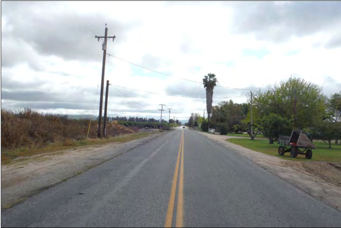
Figure 1 Project area, facing east from the western edge of the APE, showing Avenue 424 (paved).
