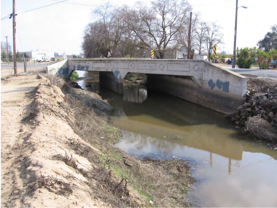
Photo 3. Avenue 424 Crossing with Flow. Looking South
