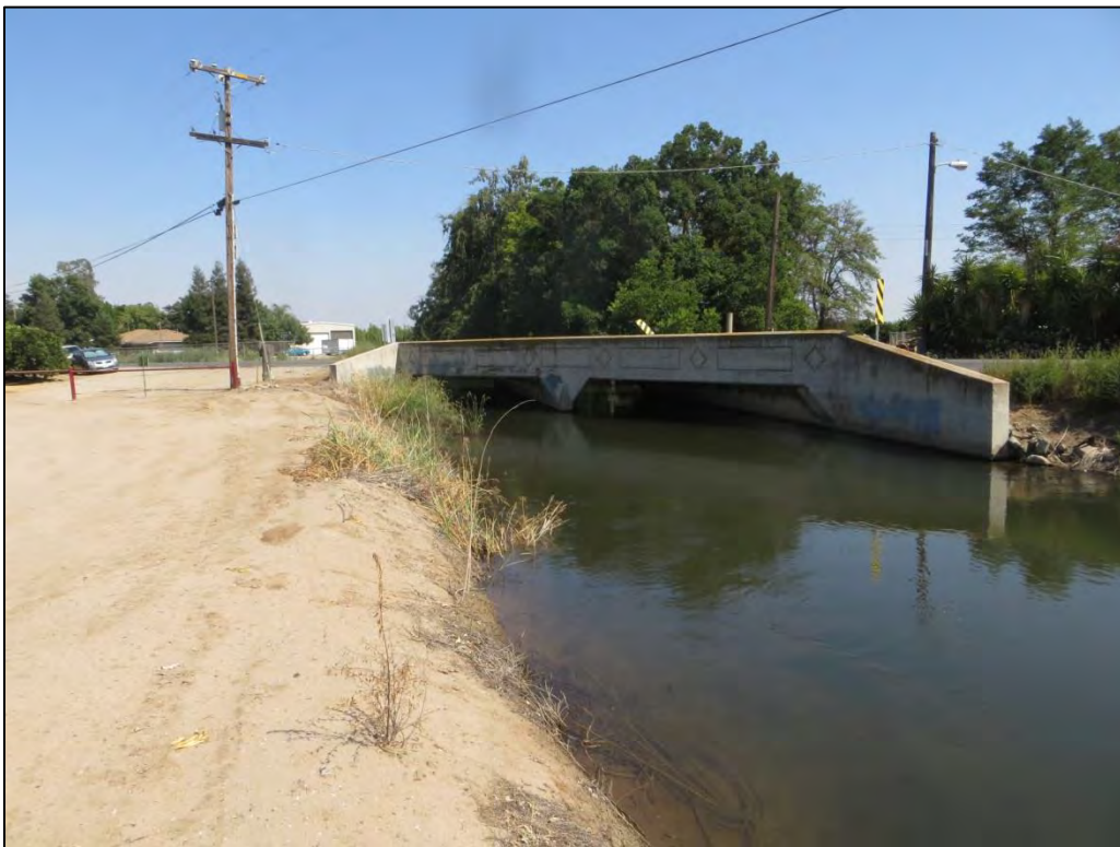
Figure 4. Bridge and canal, upstream of the bridge, facing south
