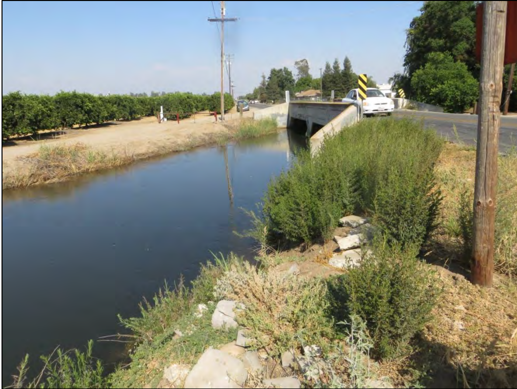
Figure 9. Canal, upstream of bridge, facing east
