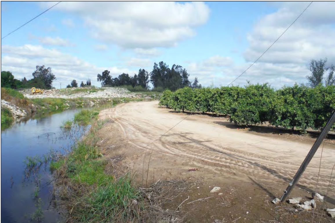
Figure 3 Survey conditions along the northeast quadrant of the APE; view of the permanent easement facing northwest.
