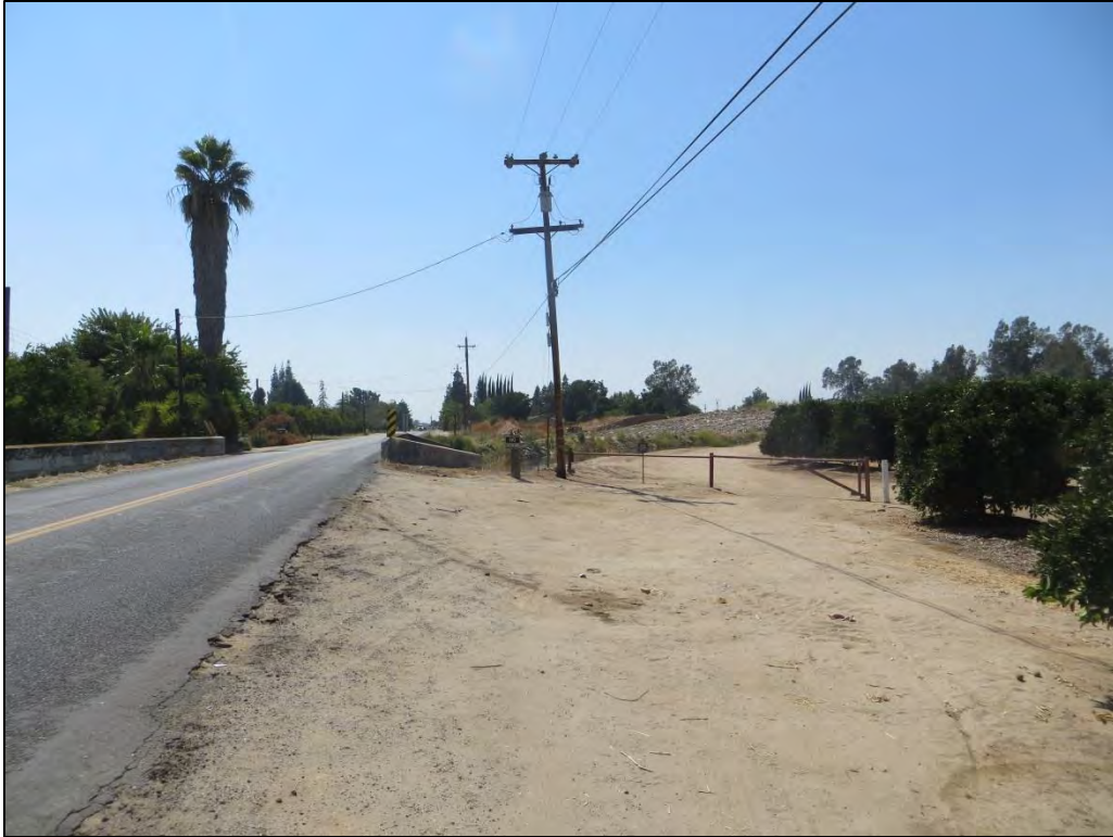
Figure 3. Avenue 424, from east of bridge, facing west
