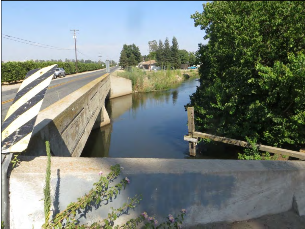
Figure 7. Bridge, downstream, facing east
