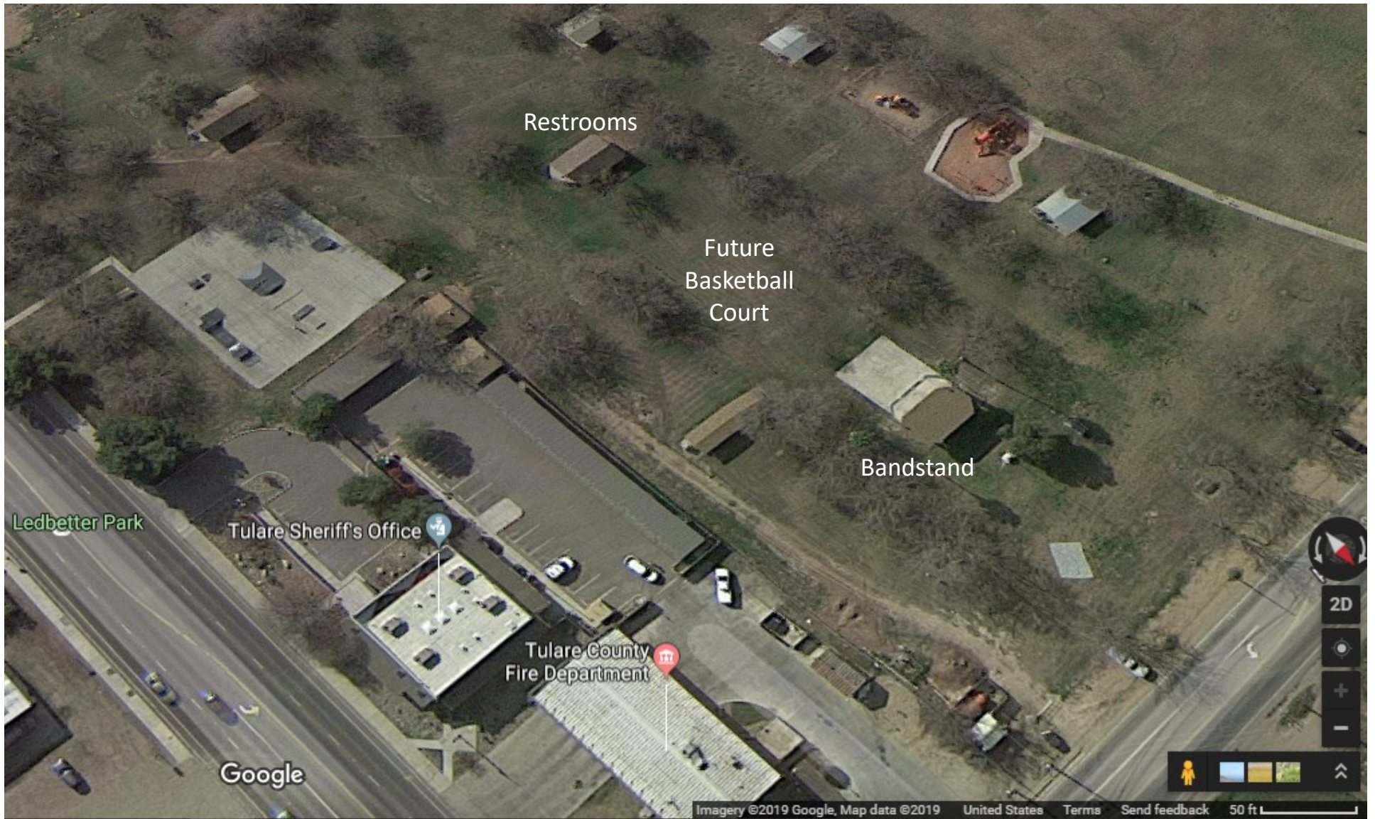
Ledbetter Park, looking southwest from the intersection of State Route 63 (Road 128) and Avenue 408. The basketball court will be constructed in the open turf area between the restrooms and the concrete slab at the front of the bandstand. The proximity to the sheriff's substation and fire station will facilitate supervision.
