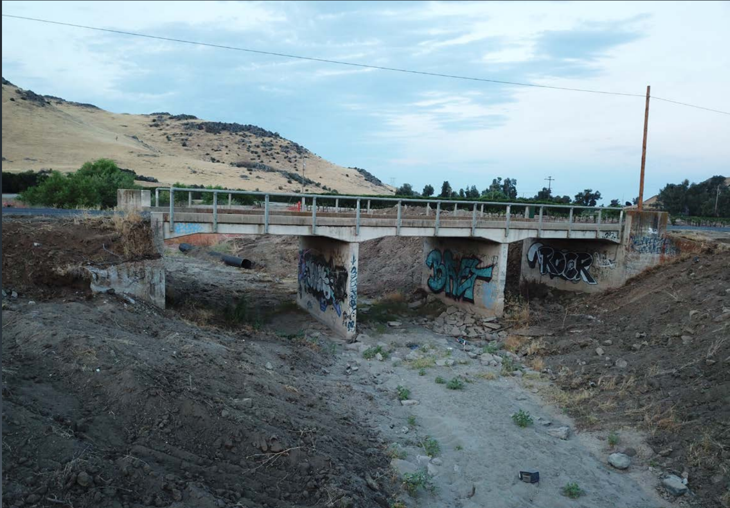
D129 over Sand Creek Bridge Project - Before
